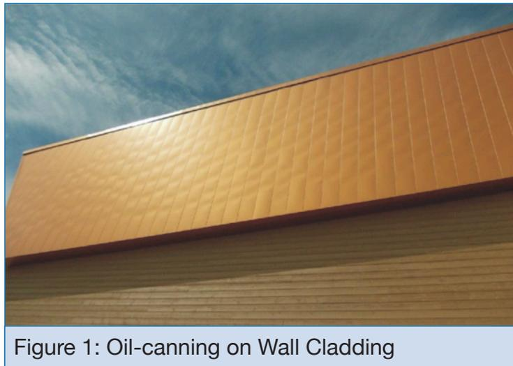
Figure 1: Oil-canning on Wall Cladding
